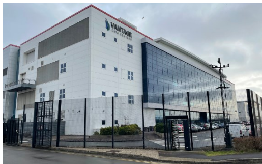
Figure 5: The CWL11 data centre
